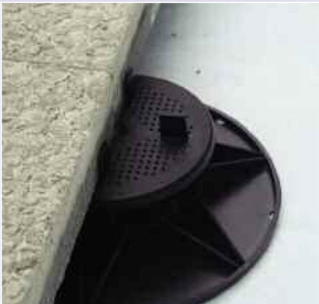
The major advantage of using support pads is that no mechanical fixings are required.
