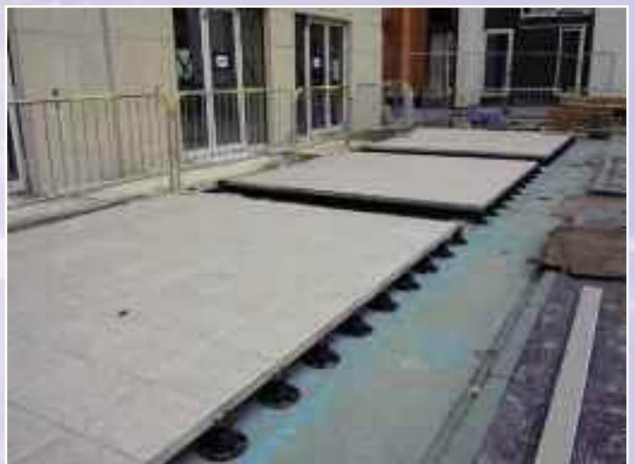
The adjustable supports are ideal for areas where a seamless terrace or walkway is required but the concrete has been cast with multiple steps or ridges. Even large differences in the height of the deck can be alleviated, creating one level across the whole area.
