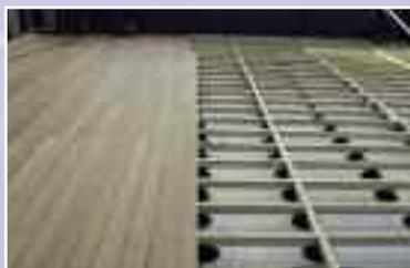
The decking layer is then fixed onto the joists using wood screws.
