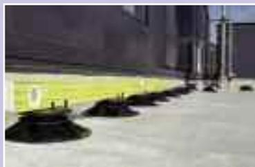
The support pads are laid out 600mm apart and adjusted so that the headpieces are level
