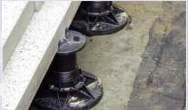
They are very easy to apply to the base plate. For the 200mm diameter base plates a simple clip mechanism fixes around the lip of the plate. All 150mm base plates have a groove inside the perimeter which slots into a series of rings situated on the slope corrector. More than one slope corrector can be applied if required as one can clip onto another very easily.
