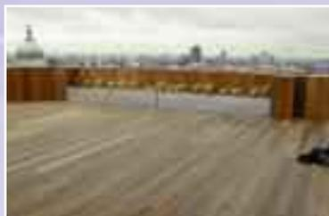
A small gap between each plank of decking should be made to help with drainage. A stunning finish can be achieved with a natural, luxurious look to the terrace. The decking runs seamlessly up to the border, planters and door threshold.
