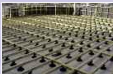
The whole area is covered by the timber joist framework right up to the edges. This frame should be able to withstand weight and vibration
