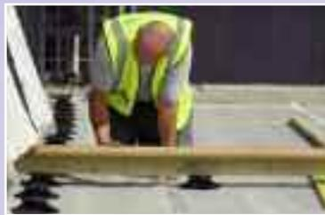
A 50mm wide joist or batten is fitted on top of the headpiece in between the lugs
