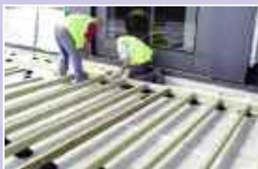
A framework of timber joists is created with the planks and cross battens fixed securely to give a strong, stable frame
