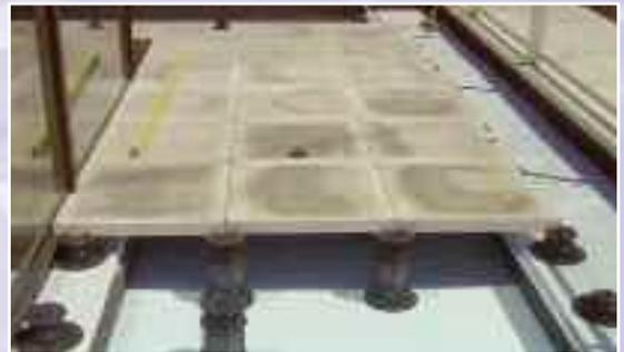
The Megapad units are made up of fixed sections (called Towers) which click into the sheath securely, and an adjustable section on the top end of the support which holds the headpiece. The amount of height adjustment depends on the size of the unit. The taller Megapads have a height range of 100mm each.
