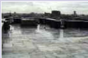
After waterproofing and insulation is installed, a geotextile membrane is loose laid on top
