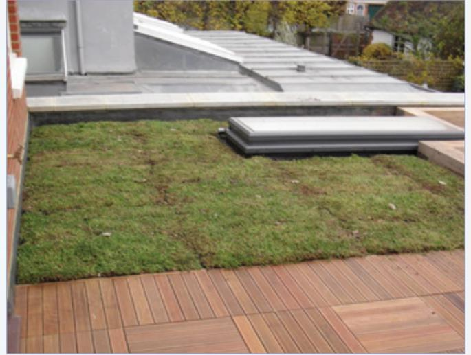
The modular sections mean detailing around objects is a simple process and clean lines are created. Hard landscaping sections such as paving and decking, mounted onto Wallbarn pedestals, can be added to the area to allow for regular access. As everything is suspended on top of the deck, drainage is uninterrupted.
