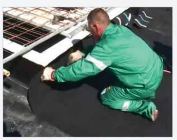
Wallbarn Protecto-mat is ideal for vertical surfaces and detailing and can be easily cut using a sharp knife and shaped around particular corners and details.
