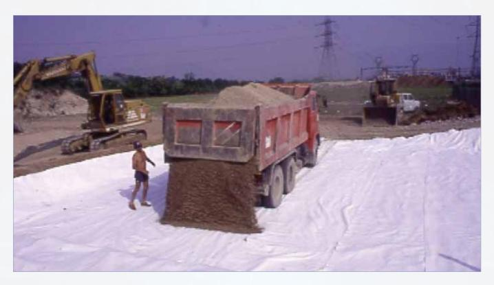
Its soft, cushioning properties mean it can be placed onto rough areas to prevent sharp objects from passing through into the system above but still allow the passage of water. This means sealing and waterproofing sheet membranes can be installed above them without the risk of ground settlement causing any damage above.
