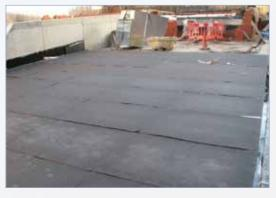
Protecto-board can be left exposed for a certain period of time and will not delaminate when coming into contact with water.
