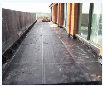
It is very easy to handle and apply. The boards will tolerate high temperatures so can be laid directly into hot melt waterproofing membranes without issue. The boards can be spot bonded or fully bonded to the membrane beneath or loose laid and taped around the edges of each board. They can also be mechanically fixed to the surface beneath.
