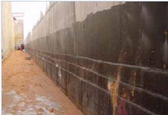
Bituminous Protecto-board can be used as a permanent layer, part of the waterproofing system, or as a temporary protection which is removed after the passing trades have finished.
