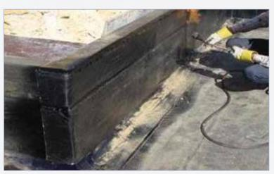
The material is supplied in  $1m \times 2m$  sheets and packed onto double size pallets for effective movement to site. The pallets hold  $200 \times 3mm$  sheets or  $100 \times 6mm$  sheets.
