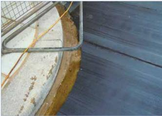
The boards are flexible enough to manipulate and shape around particular details. The sheets can be scored or cut with a sharp knife to fit around corners and multiple layers can be fitted on top of one another to give extra protection on susceptible areas.
