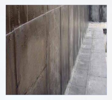
Protecto-board is lightweight and easy to handle. It can be used on both horizontal and vertical applications and can be bonded directly onto the waterproofing membrane without interfering with the seal. It is covered one side with a polyethylene film, meaning the bitumen does not bleed during storage or after application onto other surfaces.
