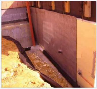
As the water drains vertically down the membrane, it is channelled through the geotextile fabric and into a perforated pipe.
