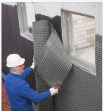
Protecto-drain 8 is available as a standard 550gsm membrane. Special lightweight or heavy duty versions are also available.
