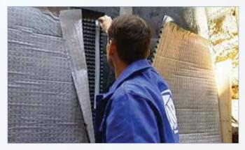
Being bitumen based, the tape has very strong adhesion and is waterproof, not becoming affected by damp. It can help maintain the waterproofing integrity of the plastic membrane.
