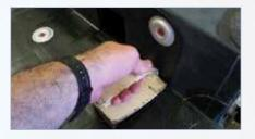
Although the flange is not perforated, the surface has a textured surface so the waterproofing or adhesive will still grip onto the material, ensuring a good bond.
