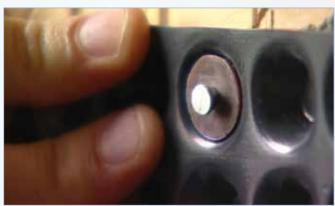
For longer fixings specialised anchors made from metal or plastic can be used to pass through the membrane. The plastic anchor has a ridged shaft to maintain a strong bond into the structure.
