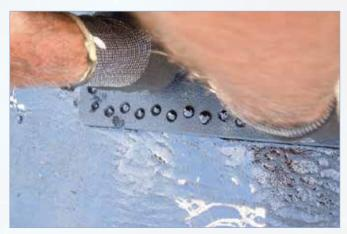
The outlet is then placed on top of the patch when the bitumen is still tacky and pressed into it firmly Some of the bitumen oozes through the perforations.
