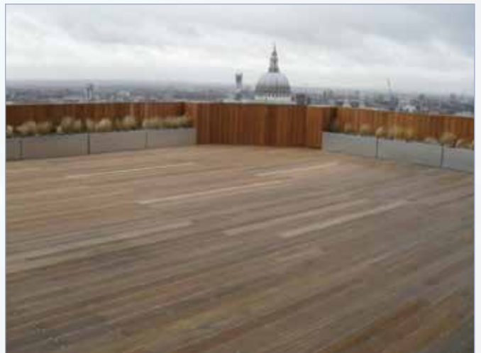
Yellow Balau tropical hardwood fixed to treated softwood joists – office development, City of London
