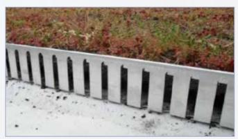
Where there is an exposed edge with no parapet, the perforated aluminium angle can be used to provide an edge to the green roof itself. It is recommended that the angle is mechanically fixed to the deck in some way. The pebbles are then installed the other side. This ensures free flow of drainage water.
