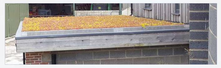
The profile is right angled, so it can sit underneath either the M-Tray® or the pebbles and be weighted down sufficiently.
