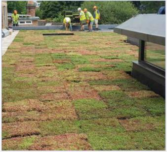
3. The edges should be filled with a border of washed riverstones, in accordance with the GRO code of practice. Objects such as roof lights and cables should be surrounded with riverstones to prevent root invasion and act as a fire break.
