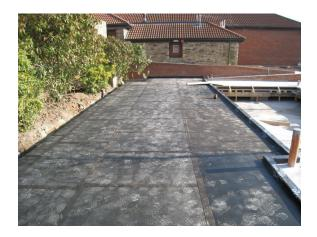
Protecto-board is loose laid over the compatible membrane and either covered straight away with another layer, pressed into the still tacky heated membrane or spot bonded using compatible adhesive on part of the membrane. Protecto-board can also be installed by butting the boards together and covering the joints with strong bitumen tape. Protecto-board is particularly useful for cutting and shaping around details such as outlets and upstands.
