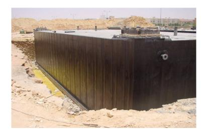
Protecto-board can be fixed to the vertical plane by torch bonding to the surface beneath, mechanically fixing or by securing with strong double-sided bitumen Protecto-tape. This is useful for temporary protection, where areas need to be guarded against following trades, and the boards taken up at a later date if required.
