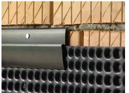
C An edge profile is used as the top finishing element on dimpled and drainage membranes.
