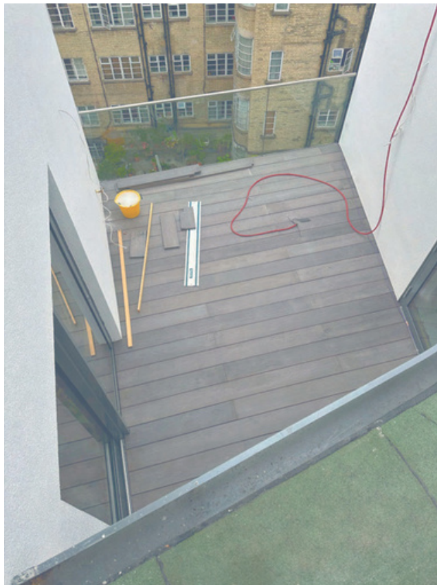
PROJECT: PENTHOUSE · LOCATION: KENSINGTON · MATERIAL: FIRE DECK QUARTZ GREY
